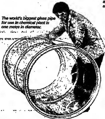
The world's biggest glass pipe for use in chemical plant is one metre in diameter.
